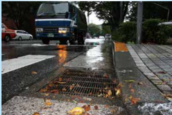
A drained road
