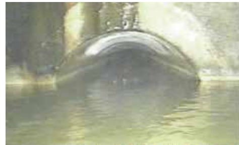
Old trunk sewer with high water level in pipe (Kotta trunk sewer)
