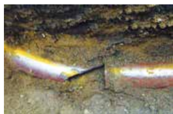
<Replacement of damaged installation pipe with high-impact rigid PVC installation pipe>
