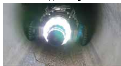
<Internal pipe investigation>
