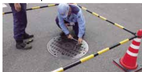
<Inspection of manhole covers>
