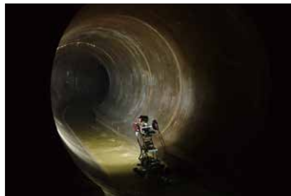
Pipe Inspection Using TV Cameras
