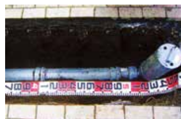
<Replacement of damaged installation pipe with high-impact rigid PVC installation pipe>
