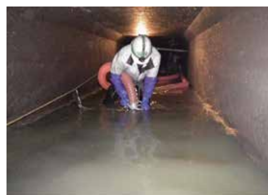
<Cleaning inside pipeline>
