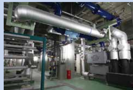
Installed air conditioning system using sewage heat to provide heating and cooling for the entire upper space building
