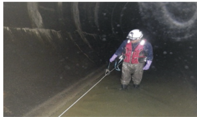
Trunk sewer inspection (Kita-Tama Nigo Trunk Sewer)
