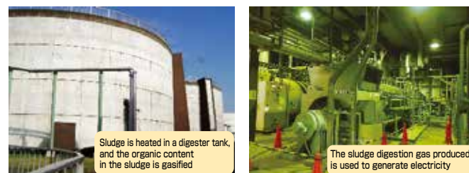
Sludge digestion gas power generation (digester tank / generator)
