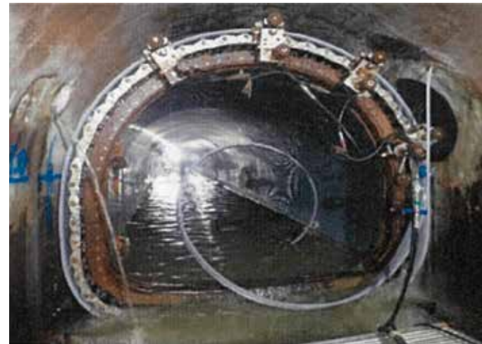
Reconstruction of trunk sewer using rehabilitation method (Yatagawa trunk sewer)
