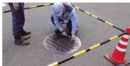
<Inspection of manhole covers>
