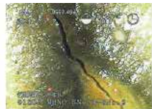
↑ Sewer damaged due to aging *Enlarged photo
