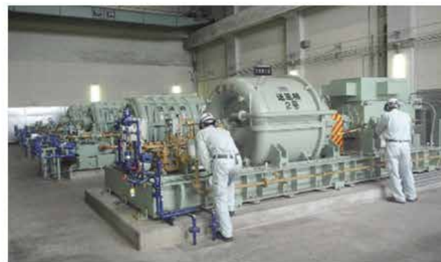
Blower inspection (Kita-Tama Ichigo Water Reclamation Center)
