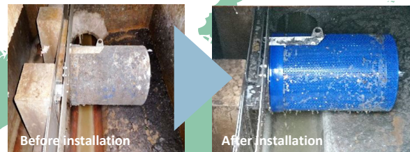
Photo1: Mechanical screen status before and after installation
