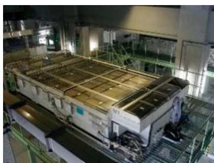
Toubu Sludge Plant Belt-type sludge thickener (Energy-saving equipment)
