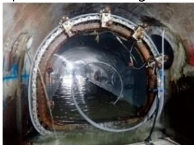
Reconstruction of trunk sewer by rehabilitation method (Yatagawa Trunk Sewer)
