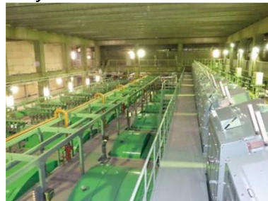
Rebuilt mechanical equipment of grit chamber
