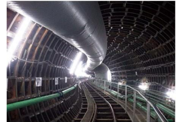
Construction of wastewater system trunk sewer (Senkawa Reinforcement Trunk Sewer)
