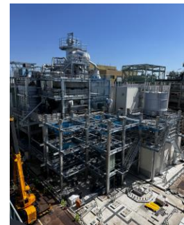
Energy Self-Sufficient Incinerator under Construction (Nanbu Sludge Plant in Tokyo)
