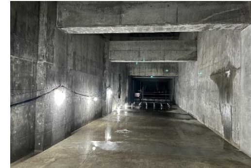
Storage Facility within Oji No.2 Pumping Station under Construction
