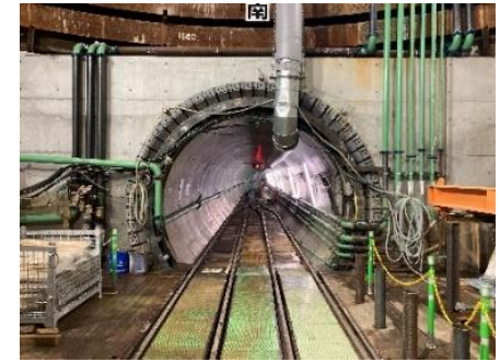
Trunk Sewer for Rainwater in the Upstream of Karabori River under Construction Approximately 20 meter below the Ground Level
