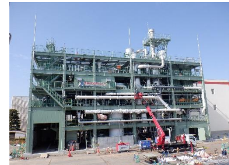
Energy Self-Sufficient Incinerator under Construction (Kita-Tama No.1 Water Reclamation Center)
