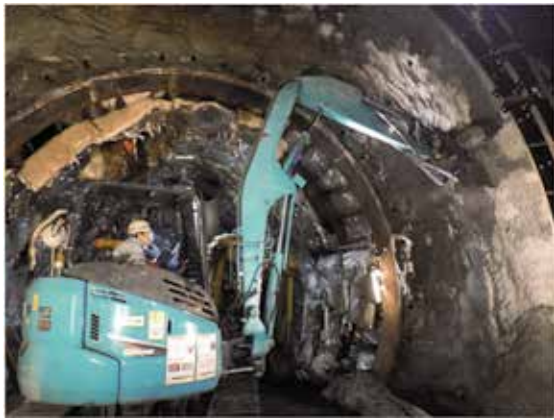
Fig.12 Frozen soil drilling
