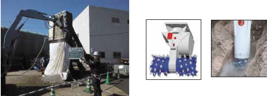
Fig.20 Test run of frozen soil excavation machine and cutting attachment
