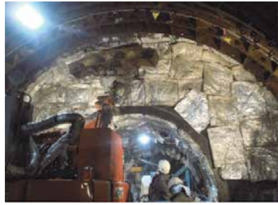
Fig.13 Segment assembling
