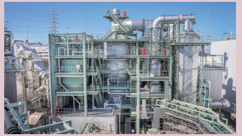
▲ Sludge incinerator
