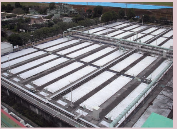
▲ Top of the storage tank (north side)
