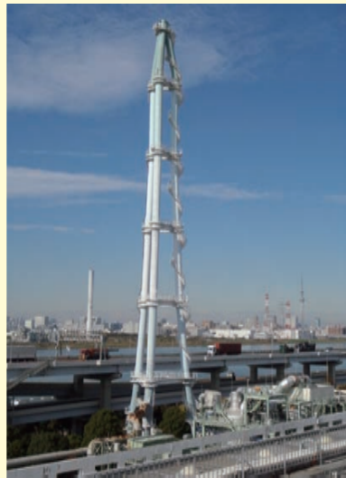
▲The smoke stack appears to be sucked into the blue sky.
