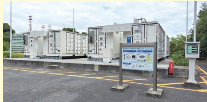
▲ NaS Battery in Sunamachi WRC
