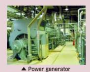
Water Treatment Plant Hot Water Power Generator Digester Digestion Digestion gas is used as Digestion Microorganisms gasify lel to generate electriciorganic substances in ty. The electricity is used the sludge. in wastewater treatment plants. Waste heat from generators is used to produce hot water to heat Gas Holder digesters. Digestion gas is stored.
