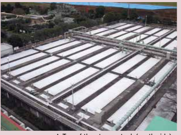
▲ Top of the storage tank (north side)
