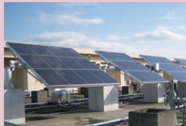
▲ Single-axis tracking type photovoltaic cell
