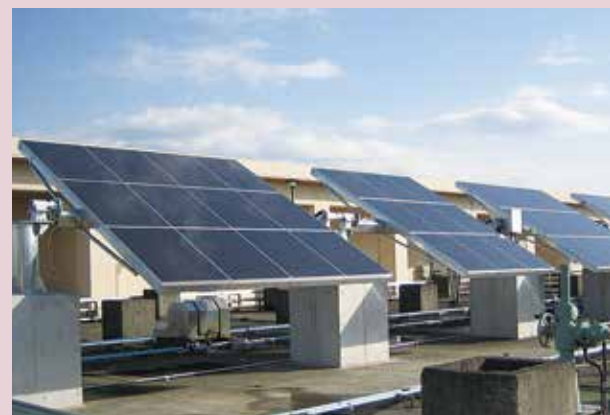
▲ Single-axis tracking type photovoltaic cell
