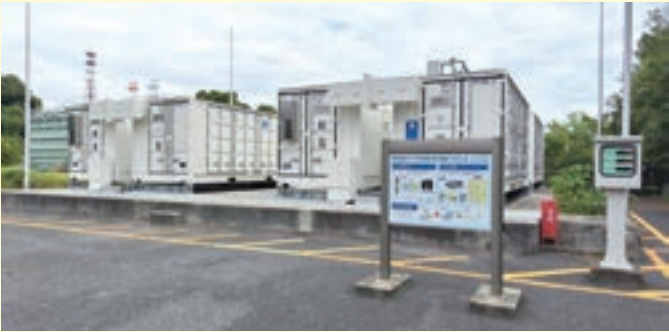
▲ NaS Battery in Sunamachi WRC
