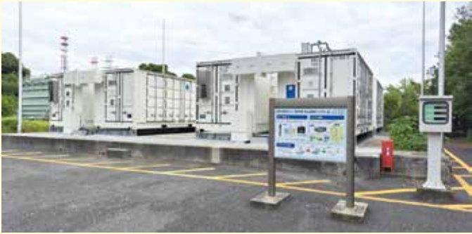
▲ NaS Battery in Sunamachi WRC
