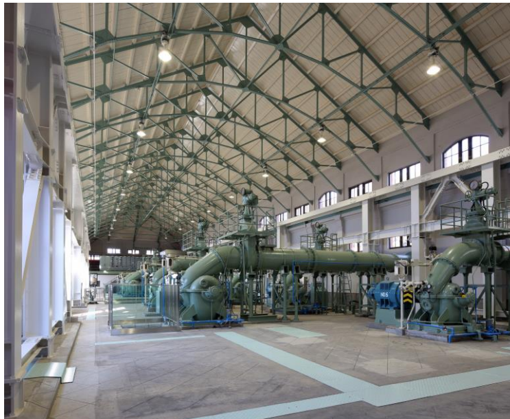
Figure2 Inside of the pump house of the former Mikawashima Sewage Disposal Plant
