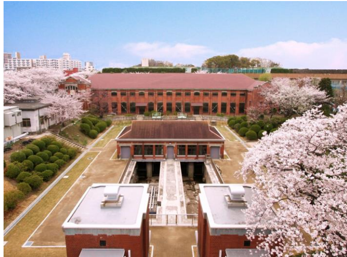
Figure 1 The former Mikawashima Sewage Disposal Plant
