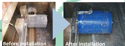
Photo1: Mechanical screen status before and after installation
